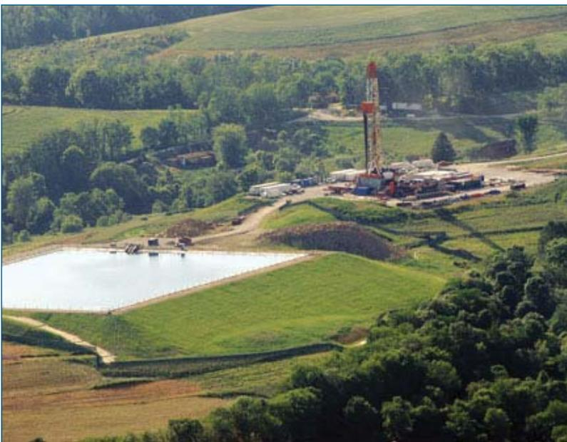
A typical drilling rig, well pad, and wastewater pond for a deep oil and gas well.
