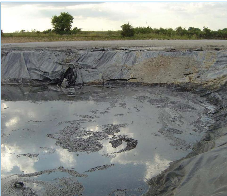
Oil and gas companies usually store the fracking chemicals, drilling mud, and other wastes in ponds on the well pad.
